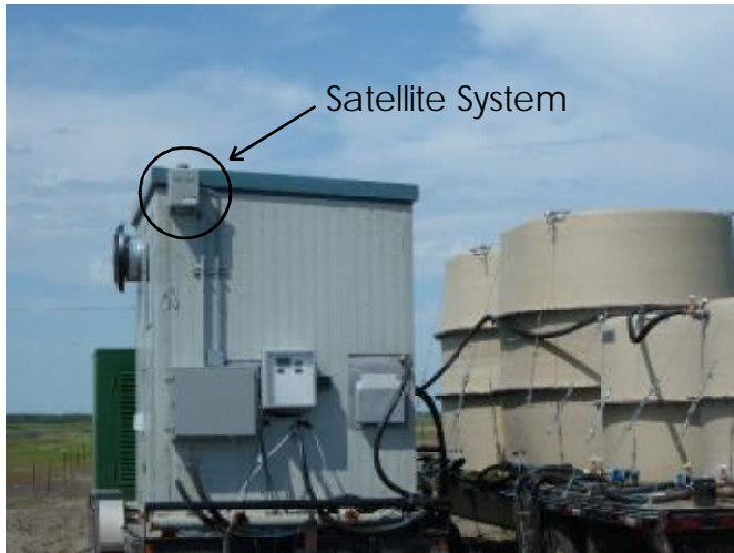
Reliable remote monitoring of tank levels, pressures and temperatures in Western Canada's oil fields saves time and money.
